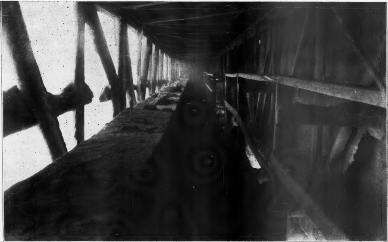
The Screw Conveyor Which Formerly Carried Cement
